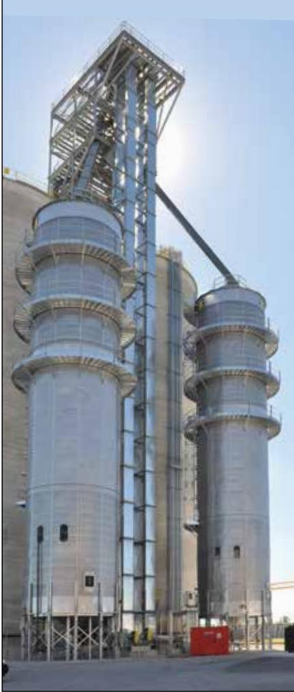
*A pair of 4,700-bph Zimmerman grain dryers are serviced by Intersystems 20,000-bph wet and dry legs enclosed in a LeMar support tower.*
