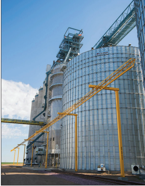
Kennebec terminal features, from left, slipform concrete storage, 80,000-bph C&A bulk weigh loadout scale housed inside the slip, 10,000-bph Zimmerman tower dryer, two Chief corrugated steel tanks, and Warrior support tower and catwalks.
