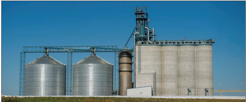
The new Wheat Growers rail terminal at Kennebec, SD has a storage capacity of a little over 4 million bushels in a combination of slipform concrete, steel, and flat storage structures. Photos by Greg Latza, PeopleScapes Publishing, Sioux Falls, SD.
